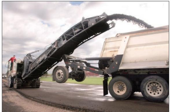
Workers from Bryco Asphalt Milling grind up the asphalt athletic track Friday morning at Casa Grande Union High School. Five inches of asphalt was removed so the track can be refurbished.
