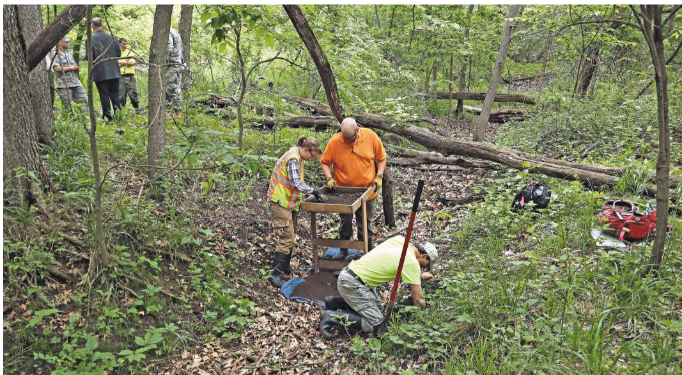
Pat Hashman digs the earth as his colleagues from Wapsi Valley Archeology, Owen Reese and Anrea Einck, sift through a load of soil on Wednesday while they all work in a recently discovered World War I-era training trench at Camp Dodge.
