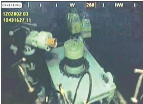
This image taken from video provided by BP PLC at 3:13 p.m. Thursday shows that oil has stopped flowing from the new 75-ton cap atop the site of the Deepwater Horizon oil spill in the Gulf of Mexico.
