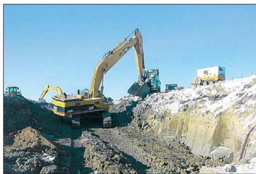
A truck prepares to unload concrete into the bucket of a backhoe carrying the concrete to workers from S.R. Weidema of Maple Grove. The workers were completing construction of the interceptor sewer line leading to Willmar's new wastewater treatment plant. The 5½-mile line was completed on Dec. 15, 2009, eight months ahead of schedule.
