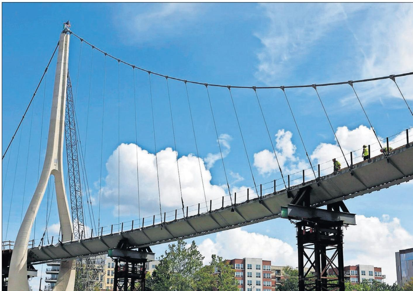
With suspension cables now in place, construction crews work on the deck of Dublin's pedestrian bridge. The bridge spans the Scioto River to connect Dublin's historic district with the Bridge Street District that is being finished. Officials have said they hope to open the bridge by year's end. Kokosing Construction Co. is building it. When complete, the bridge will be about 760 feet long.
