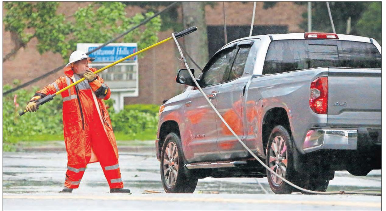
**A power line worker with Gainesville Regional Utilities uses a special insulated pole to lift a live power line off a truck Friday after strong winds knocked down a nearby tree that tore down the lines. The truck was traveling south on Northwest 34th Street near 16th Avenue in Gainesville.** [BRAD MCCLENNY/STAFF PHOTOGRAPHER]
